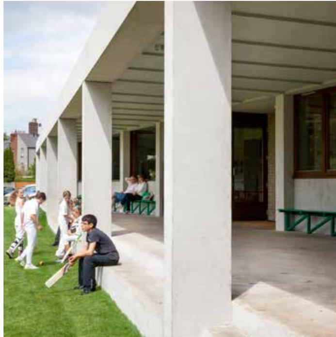
» As well as providing an open, generously scaled façade to the pitch, the move creates, through steps in section, a variety of protected viewing opportunities that layer the space. Seat-height steps are integrated into the 600mm level change on the line of the outer columns, while at a line of sight above, a series of green-painted timber benches are set to the rear of the terrace. Above these the internal windows open to provide stool-level views.
